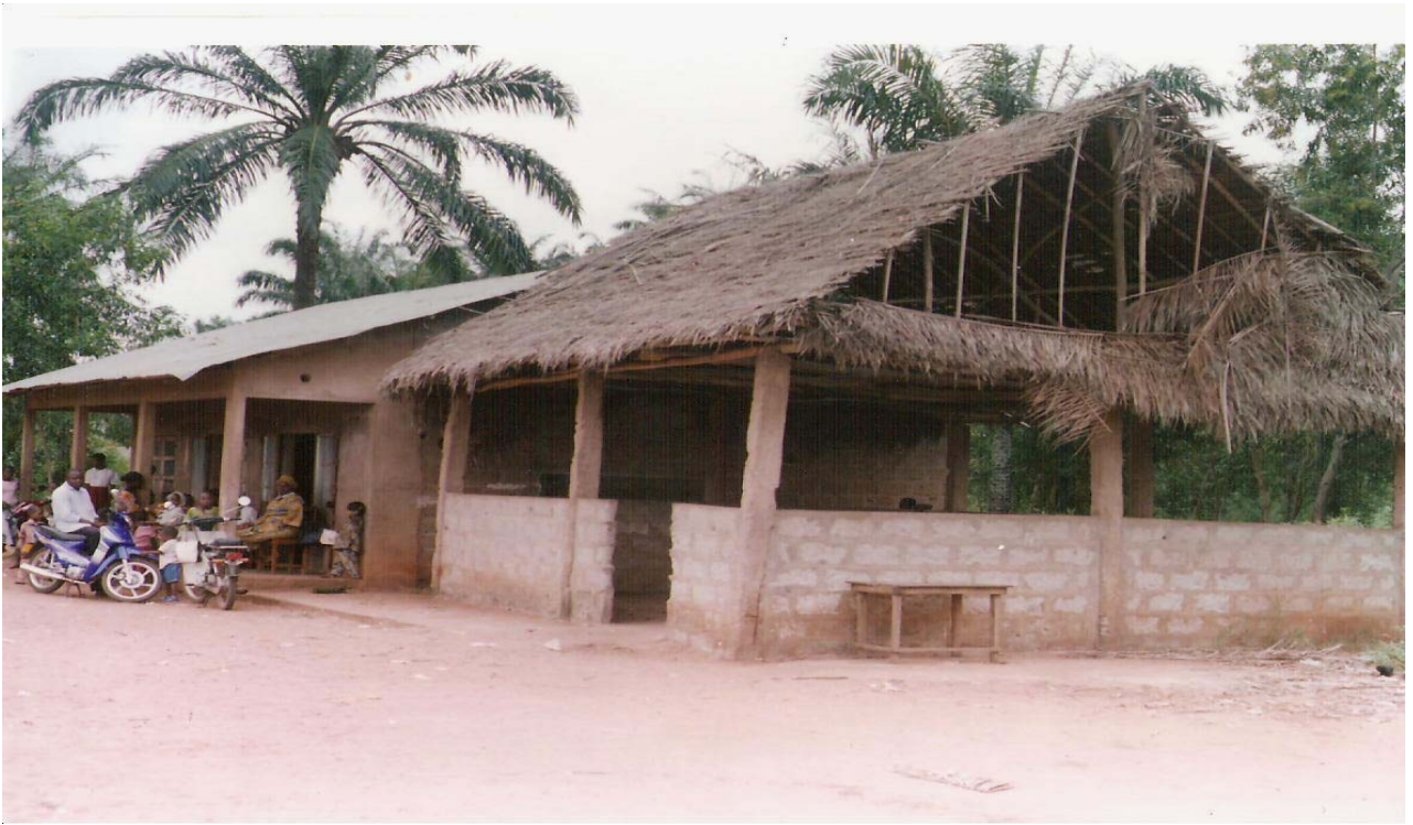
Photo 3 : EM-Vakon –Centre (AKPRO-MISSERETE)
